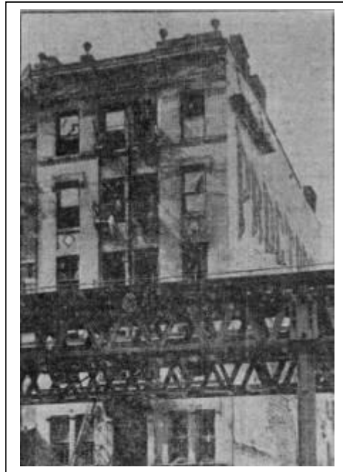
105 Allen after the fire
