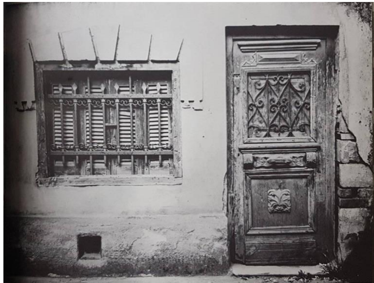
House in Baron Hirsch neighborhood in Thessaloniki before WWII These were the houses Jews were transferred to while awaiting deportation since Baron Hirsch was across from the train station.
